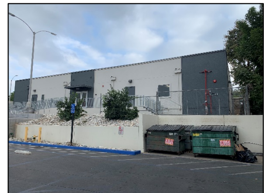
School of Medicine Modular Building
