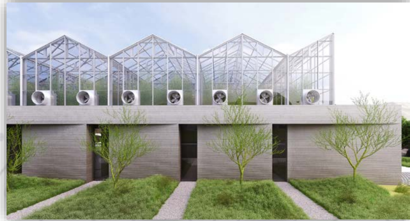
Plant Growth Environments Facility: Scheduled to be completed September 2020
