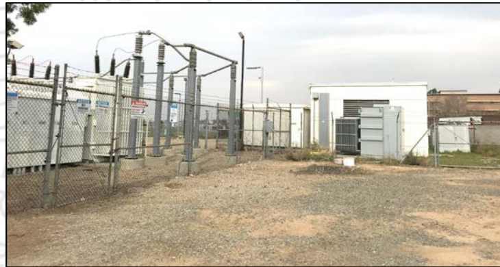
Co-Owned Electrical Utility Service
