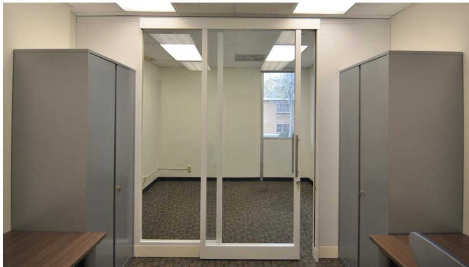
Sproul 2208 Sound Isolation Booth in construction.
