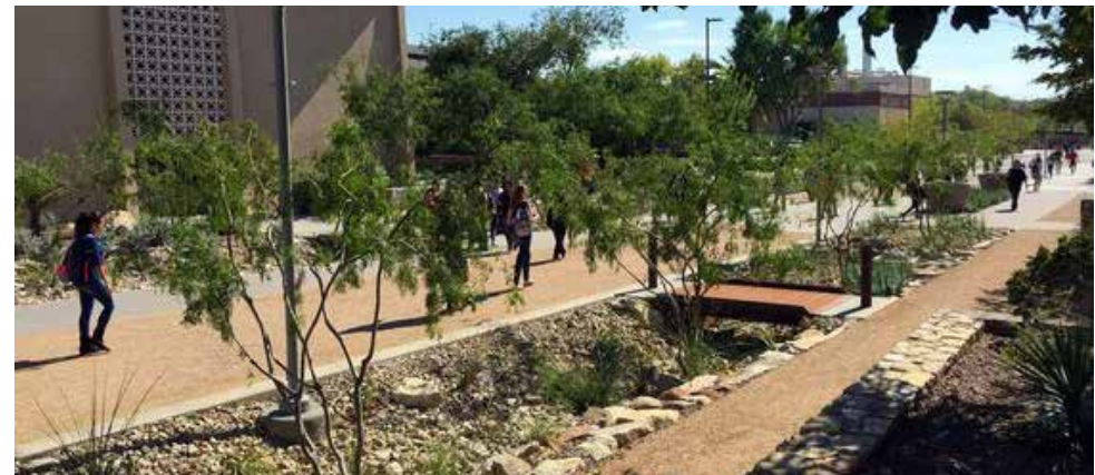
▲ Drainage clearly expressed and integrated into circulation paths to offer teaching opportunities.
